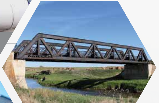
Steel Bridge Girders
